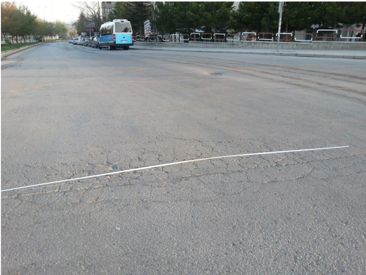
Figure 4 - Transverse Cracks
