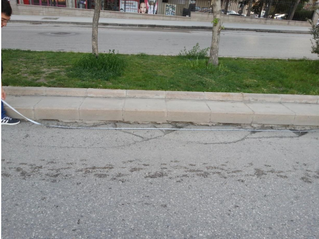
Figure 6 - Edge Cracks
