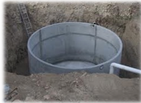
Figure 2: Underground Water Tanks
